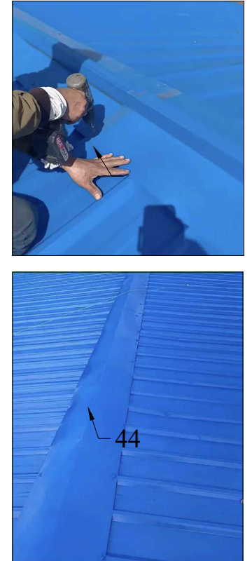
Figure 11 Installation of roof panels
